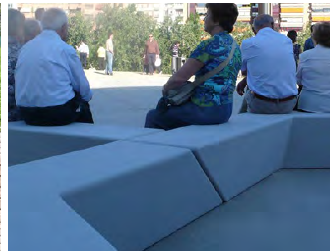
FREESTANDING PRECAST CONCRETE BENCH occurs under the 'L' Tracks Pedestrian Way
