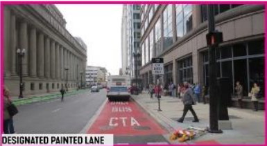
DESIGNATED PAINTED LANE
