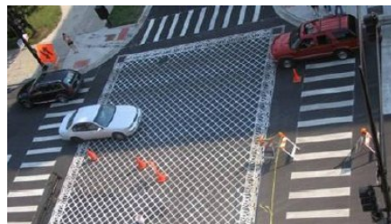
DECORATIVE INTERSECTION PAVEMENT
