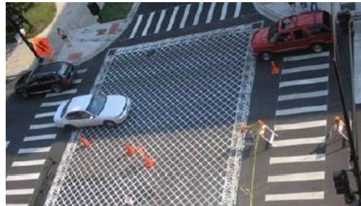
DECORATIVE INTERSECTION PAVEMENT
