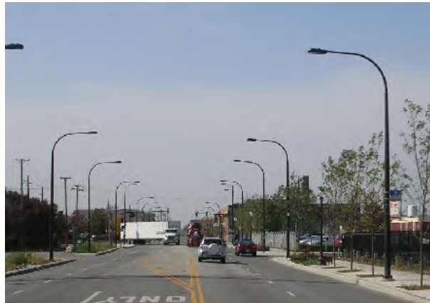
2 Davit pole replacement
