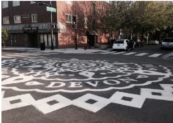
2 Epoxy embedded asphalt
