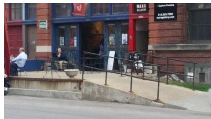
Pipe railing at Mars Gallery; steel faced curbs
