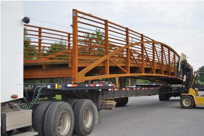
Prefab Bridge being Delivered
