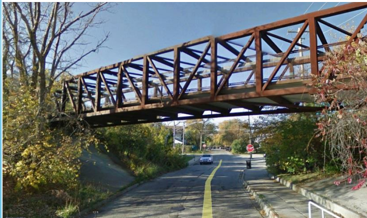
Valley Line Trail Bridge N. Rogers Ave
